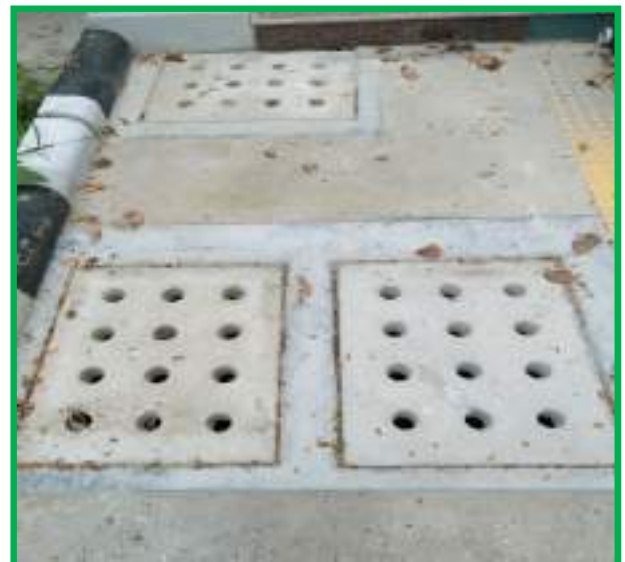
FIG 15 A PICTURES OF RAINWATER HARVESTING RAINWATER HARVESTING PITS. = 13 NOS.
