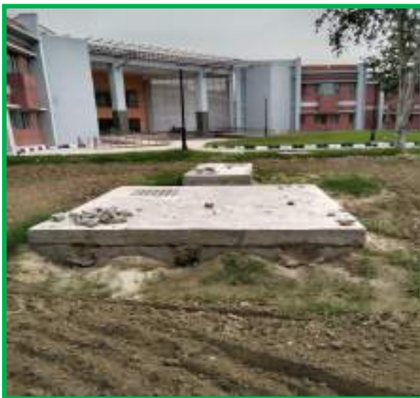
FIG 15 A PICTURES OF RAINWATER HARVESTING RAINWATER HARVESTING PITS. = 13 NOS.
