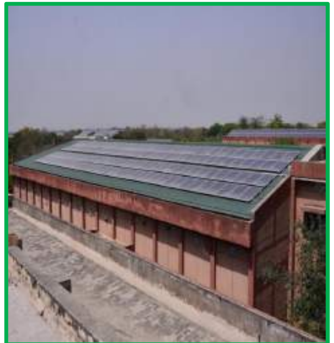
FIG. 39 SOLAR PANEL INSTALLED ON THE ROOF TOP OF BUILDINGS (SCIENCE AND MECHANICAL BLOCK)
