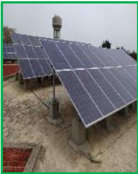
FIG 39 SOLAR PANEL INSTALLED ON THE ROOF TOP OF BUILDINGS
