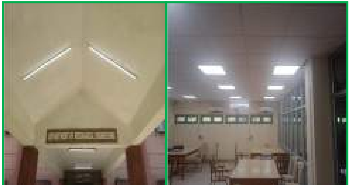
FIG- 31 LED FIXTURE IN ME ENTRANCE AND CENTRAL LIBRARY, FF (READING HALL)
