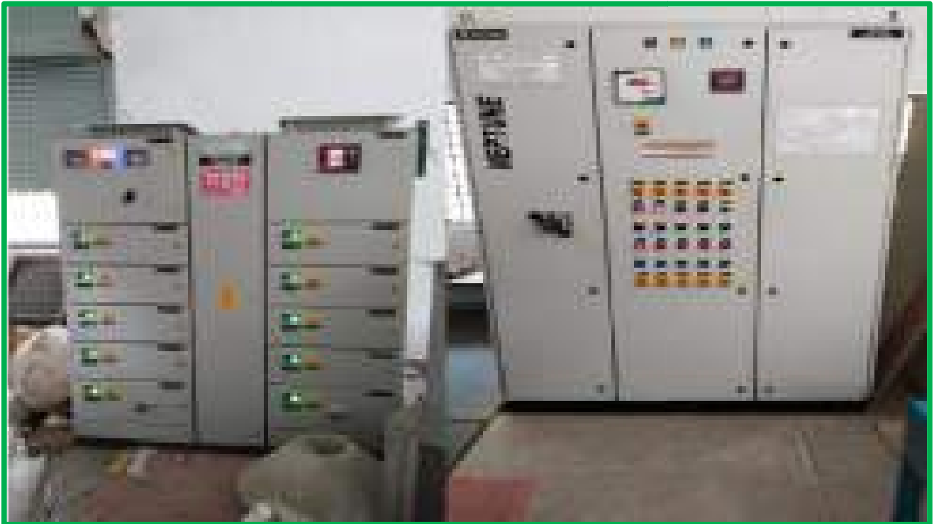
FIG. 28: APFCR PANEL AT ESS-I AND ESS-II
