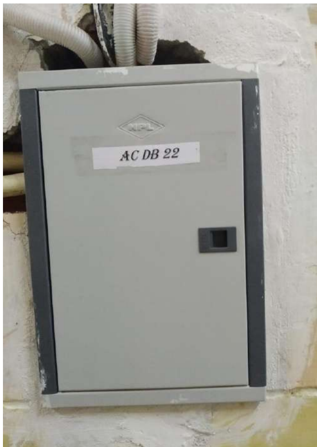
Fig.3.15. AC DB Attached in Mechanical Block for Essential and Non-Essential Load
