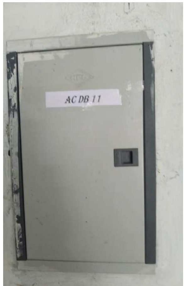
Fig.3.15. AC DB Attached in Mechanical Block for Essential and Non-Essential Load
