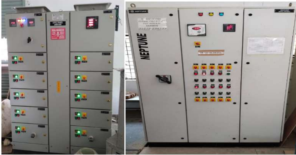
Fig. 3.1: APFCR Panel at ESS-I and ESS-II
