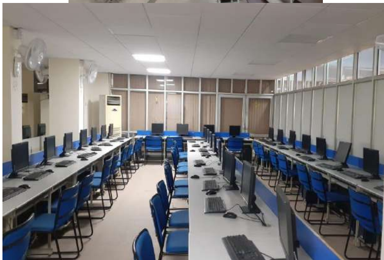
Fig. 3.7: LED Fixtures in Smart Classrooms (Science Hall 4, TF)
